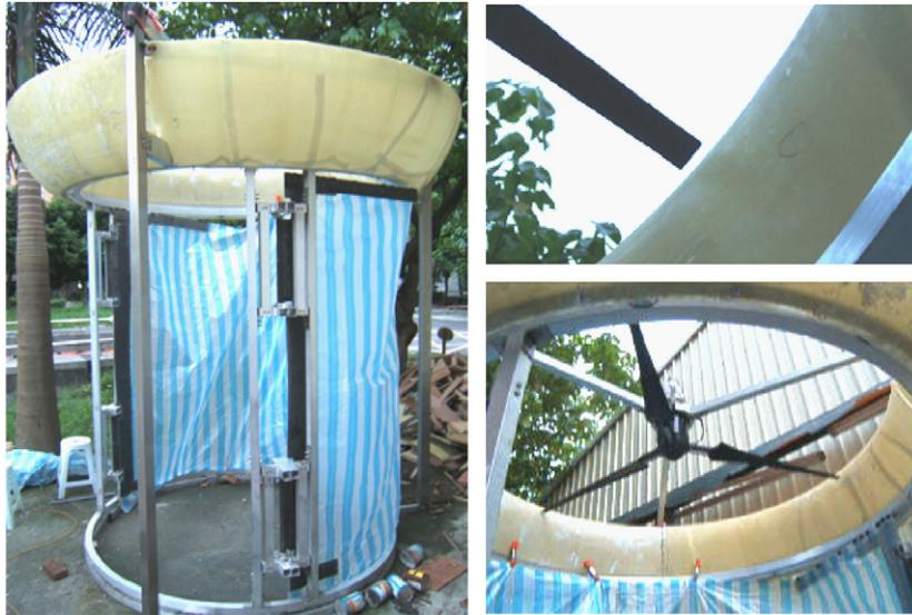
Fig. 14. Actual installation of the ducted wind turbine.
