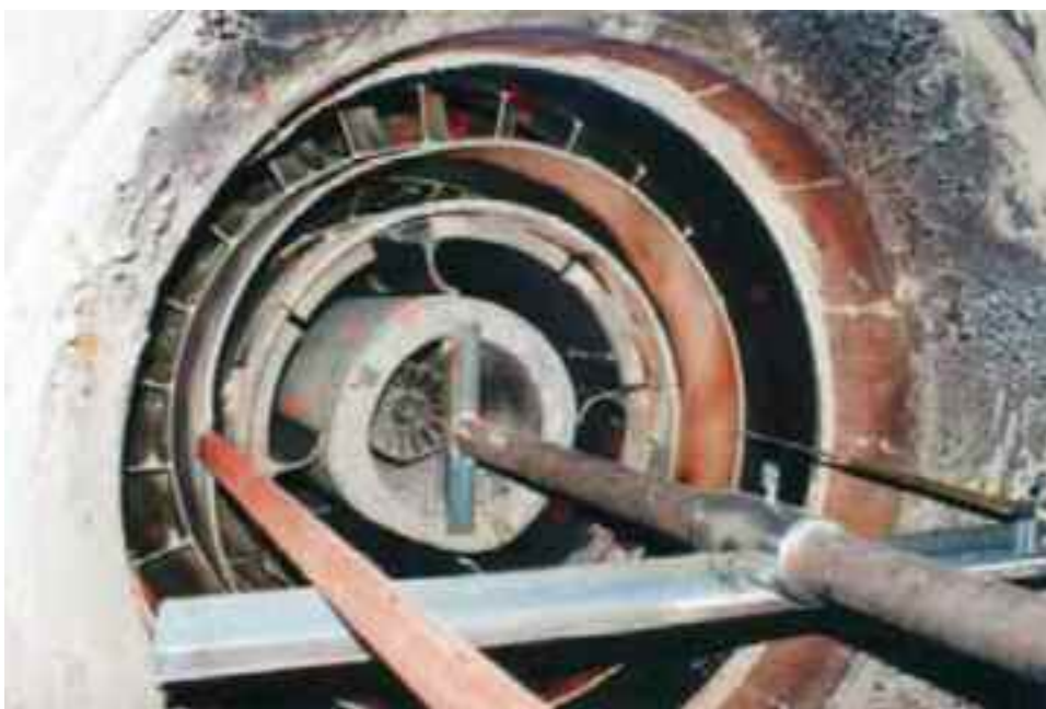
Figure 2. A Babcock Energy burner during measurements of the velocity components
