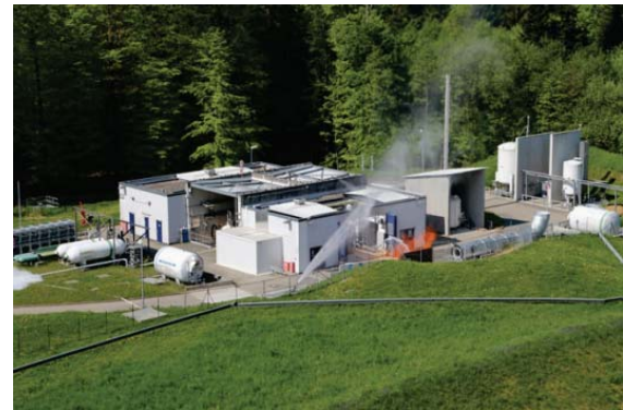
Figure 9: P8 Test Bench at DLR Lampoldshausen
