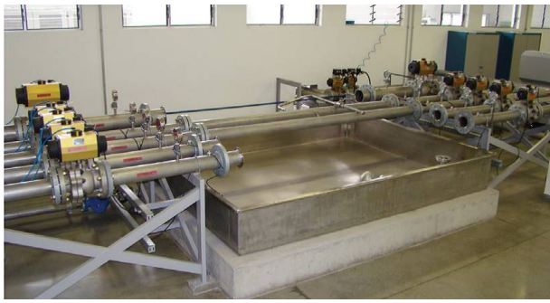
(a) Water supply of the hydraulic test bench driven by electrical pumps
