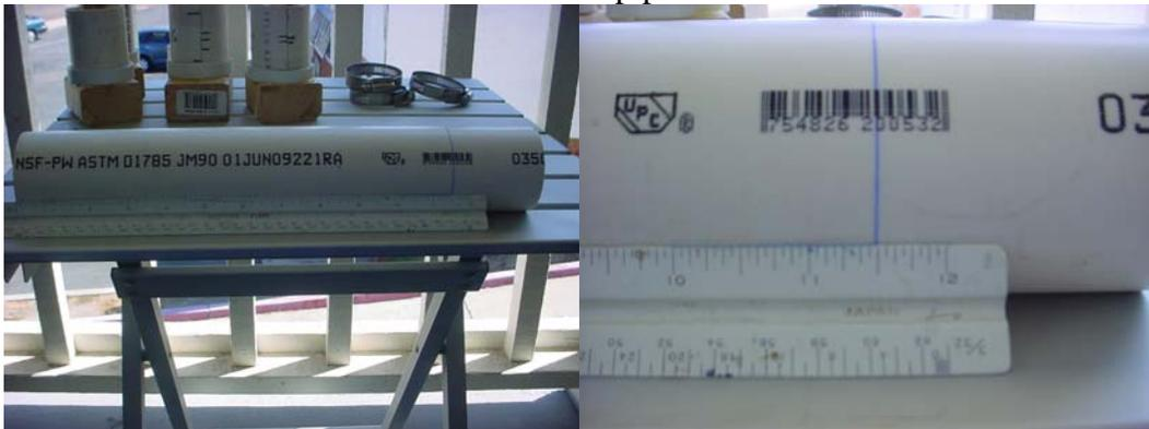
2. Measure back 1-1/8" from one end and draw a line around the pipe.
